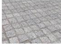
Granite sett framing surfaced areas and aiming to emphasise the heptagonal shape of the monument
